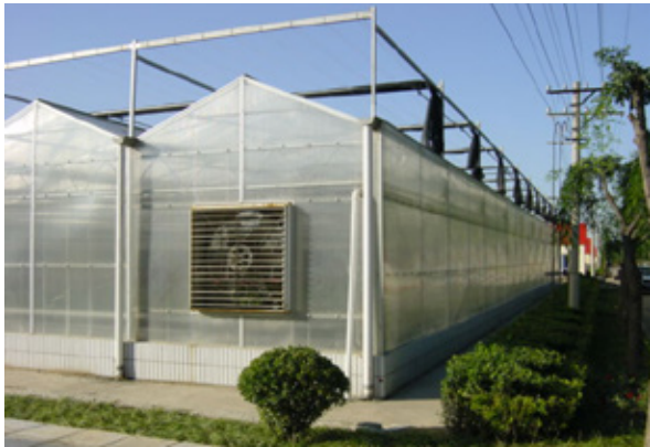
Pad/fan system and a movable outdoor screen
