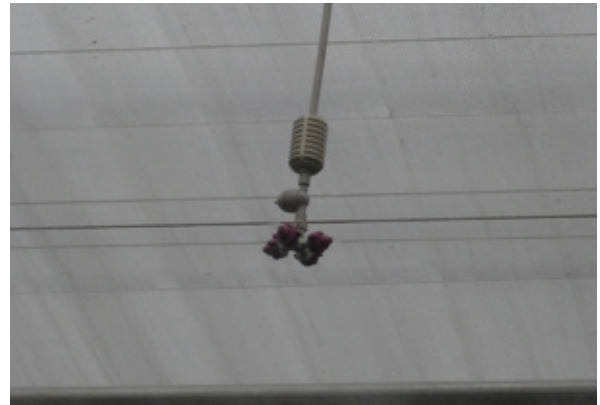
Simple low-pressure humidification
